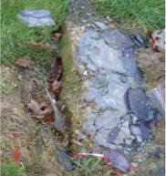
Headstones are now loose and causing a danger, these are liable to topple over with a risk of injury due to the beams breaking up. It is the cemeteries responsibility to renew the beams as the cemetery installed them.
